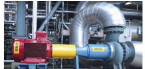
At the synthetic fiber manufacturing facility at Teijin Aramid, the Netherlands, a heat transfer pump is sealed with a high-efficiency **NMB-22P-6R-65-00** magnetic coupling. The heat transfer oil can reach temperatures of up to  $315\text{ }^{\circ}\text{C}$  ( $599\text{ }^{\circ}\text{F}$ ). The patented low eddy current gap trap keeps the power losses – and heat generation – down despite the high drive power of 45 kW.
