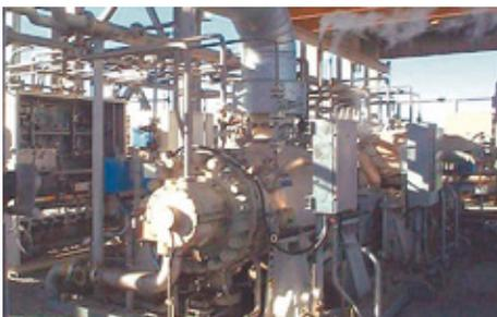
A **DGS11.1** seals a compressor in the fertilizer manufacturing facility at Incitec Pivot Limited in Australia. **Espey WD400** nitrogen-buffered carbon floating ring seals are used to seal the bearings. The process medium is a mixture of hydrogen and nitrogen. The seal is designed for frequent slow roll operation when starting and stopping the machine.
