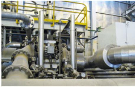
A type **DGS30** gas-lubricated mechanical seal is used to seal a compressor in BASF's synthesis gas plant in Shanghai, China. Nitrogen-buffered **Espey WD400** floating ring seals seal the bearings. The process medium is carbon dioxide. Operating conditions:  $p_1$  (dynam.) = 18.5 bar (268 PSI);  $t = 70\text{ °C}$  ( $158\text{ °F}$ );  $n = 25,750\text{ min}^{-1}$ .
