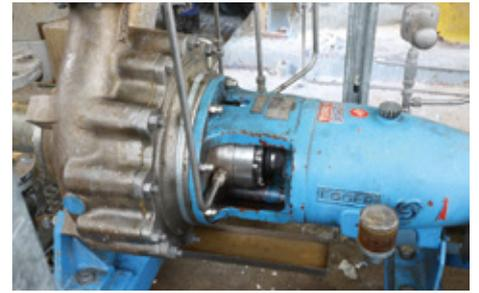
Centrifugal pumps at Polymer-Latex GmbH in Marl, Germany, are successfully sealed with **Cartex-DN** type seals. The process medium – a latex dispersion – represents a challenge for the seal. The **FLC200** flow rate control unit supplies and flushes the seal.
