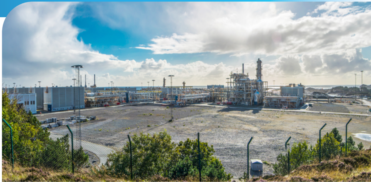
The Kollsnes gas processing plant went into operation in 1996 and has been continuously expanded since then.
